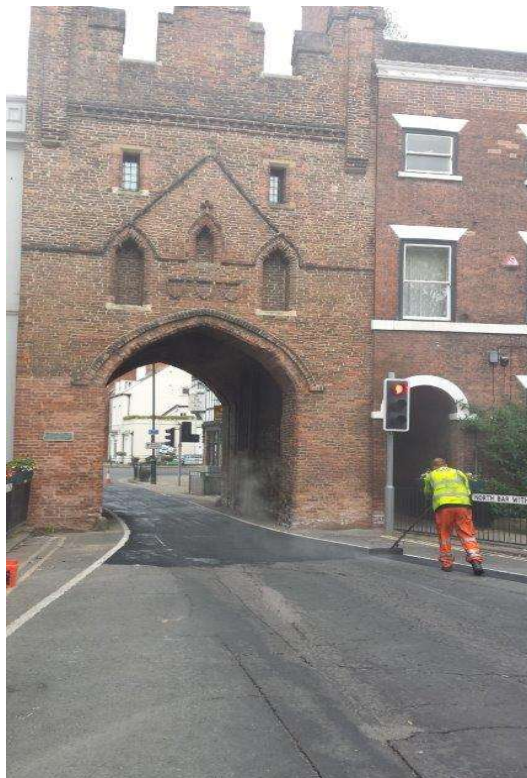
Figure 1: Work being carried out at North Bar, Beverley
