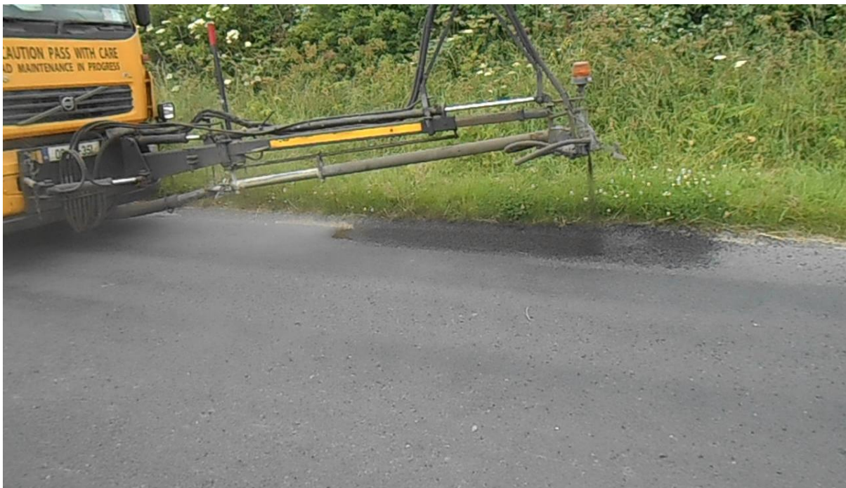
Figure 1 Roadmaster machine at work
